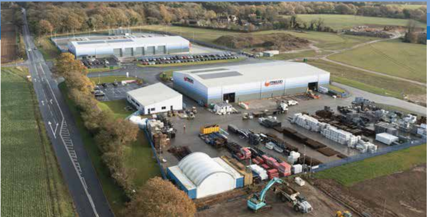
▲ Precon Products has relocated its Head Office to Unit 1
