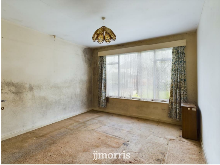
With window to the fore, storage heater.
